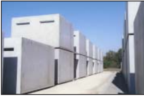
Modules staged for delivery at the GA manufacturing facility.
